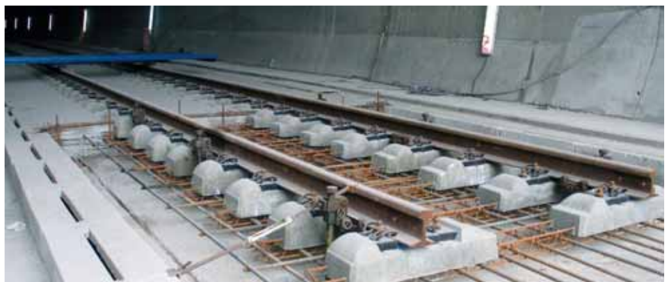
Close up of the system showing precast elements and reinforcement
