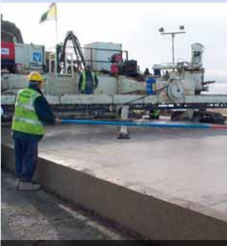
Slipforming pavement quality concrete at RAF Fairford
